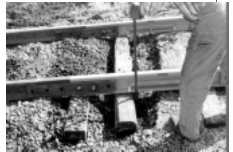
Adjusting tie spacing
