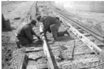
Installing Weighline rails
